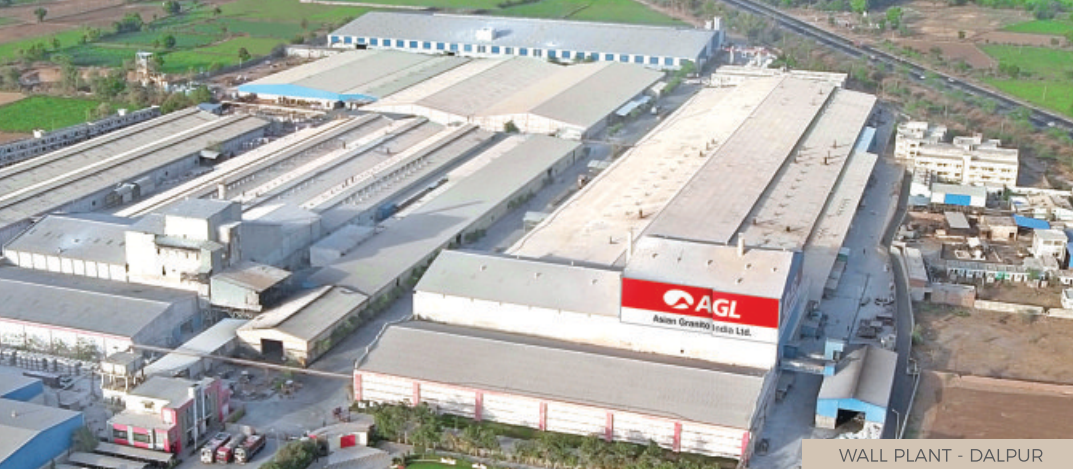
WALL PLANT - DALPUR
